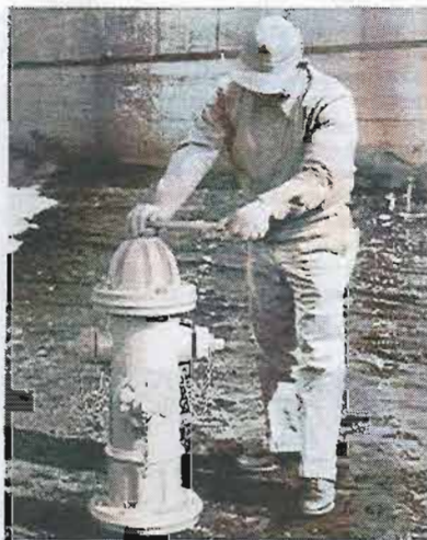
4. Tighten operating nut, turning in closing direction.
