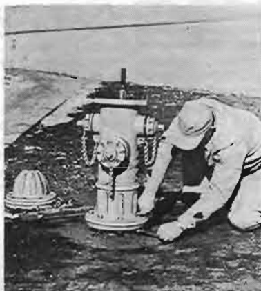
5. Place flange gasket on exposed flange of lower barrel. Place upper barrel carefully in position on lower barrel. Be sure that it is concentric with lower barrel and that gasket is centered.
