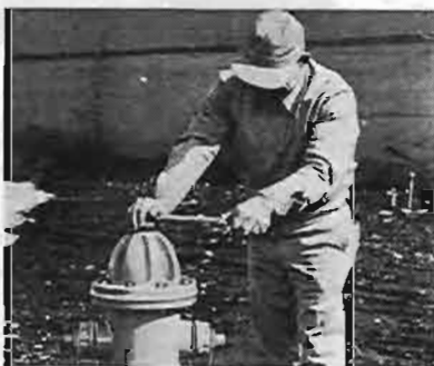
7. Replace Hold Down Nut being sure "O" Ring seals are in good condition at thread shoulder on outside of Hold Down Nut and on inside where contact is made with Operating Nut. Replace Weather Cap. Tighten bonnet bolts. Check gasket tightness by opening one hose cap slightly before opening hydrant to bleed air. Open hydrant until barrel fills with water, tighten hose cap, open hydrant fully. Check gaskets, and then turn Operating Nut to fully closed position.
