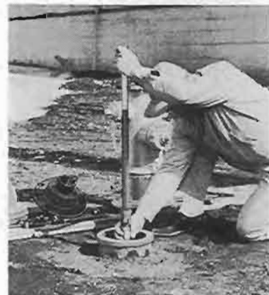
3. Remove damaged coupling and sleeve. Screw new safety stem coupling on to lower stem down against shoulder. Slip safety sleeve over lower end of upper stem section. Screw upper stem into safety stem coupling until it contacts the lower stem.
