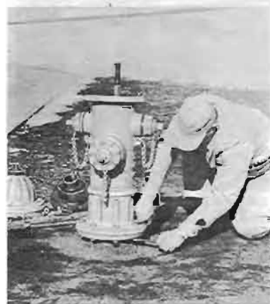
5. Place flange gasket on exposed flange of lower barrel. Place upper barrel carefully in position on lower barrel. Be sure that it is concentric with lower barrel and that gasket is centered.
