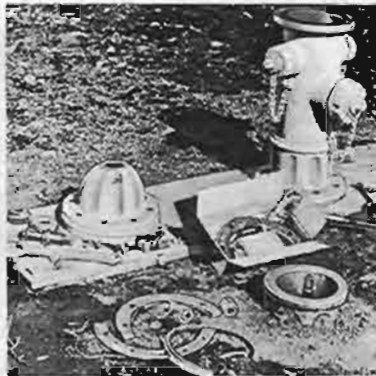
2. Unbolt and remove broken Safety Flange from upper barrel. Remove Weather Cap, Hold Down Nut and Operating Nut from bonnet. Lubricate A-24099 Brass Sleeve and slide over threaded stem end to prevent "O" Ring damage. Unbolt bonnet from upper barrel. Slide upper stem out of bonnet. Remove broken Stem Coupling from upper stem by placing a narrow faced chisel between lug part containing set screw and strike a sharp blow with hammer to break off lug. Unscrew remaining coupling part from stem or break coupling part from stem with hammer. Unscrew lower part of coupling from lower stem or break away with hammer.
