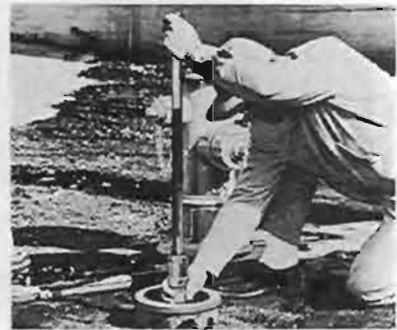
3. Draw a chalk or pencil mark on lower stem in line with tongue and a similar mark on upper stem in line with the groove. Screw new Coupling down until it shoulders on lower stem. Engage upper stem with Coupling and screw down until it contacts lower stem. Back up the upper stem just enough to line up the marks drawn on the stems. Hold upper stem stationary and rotate Coupling upward until tongue and groove lock firmly together. Tighten set screw.
