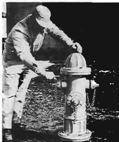
1a For hydrants without oil hole in bonnet use the following alternate procedure. Remove four bonnet bolts.
