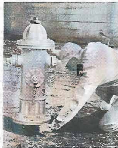
5. Tighten safety flange bolts.
