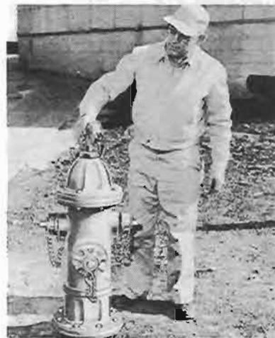
3. If oil is low, add oil using a small funnel or oil can in oil hole. (For hydrants other than SR, check level again with dip stick. Repeat until oil is up to mark on dip stick.) Replace filler plug in oil hole.
