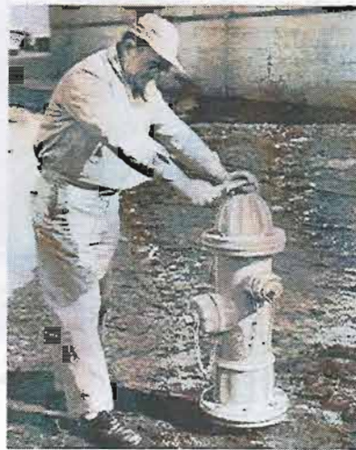
2. Turn operating nut slightly in the opening direction to relieve compression between barrel sections.
