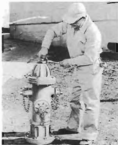
1. For all hydrants having oil hole in bonnet, remove filler plug and check oil level.
