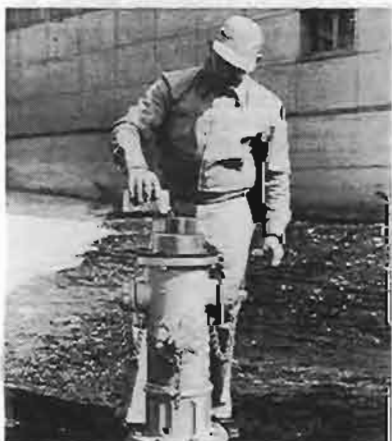
6. Check stuffing box gasket. Lubricate A-24099 Brass Sleeve. Slide Sleeve over threaded area of stem to protect "O" rings from damage by threads. Place stuffing box plate in position and bolt to barrel. Remove Brass Sleeve. Pour Mueller Hydrant Lubricant into oil reservoir until THREE-QUARTERS of an inch from top.
