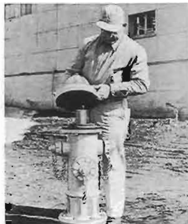
3a. Remove bonnet. Properly adjust packing if not "O" ring type.
