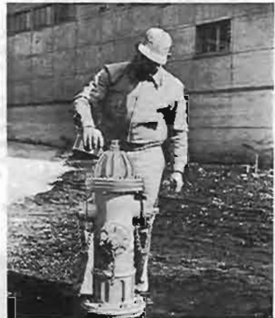
6. Check bonnet gasket. Attach the A-24099 Brass Sleeve, if it had been removed, to upper stem and lubricate outside to protect "O" Ring seals from thread damage. Place bonnet onto upper barrel and assemble bonnet bolts only hand tight. Remove Brass Sleeve. Reassemble Operating Nut and remove Oil Plug in side of bonnet. Pour Mueller Hydrant Lubricant into oil reservoir until it is level full with Plug. Replace Oil Plug.
