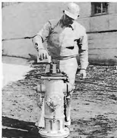
4a. Replenish Mueller Hydrant Lubricant, if necessary, to within three-quarters of an inch from the top of oil reservoir.
