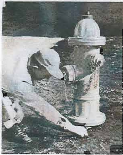
1. Loosen nuts on safety flange bolts.
