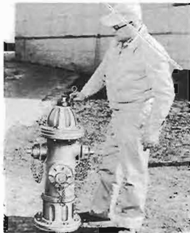
2. For sealed oil reservoir style (marked SR) oil should be level full with plug. (For other hydrants having oil hole in bonnet, insert dip stick into hole until it rests on bottom of oil reservoir.) Remove dip stick and note if oil is up to mark.
