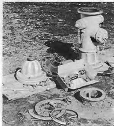
2. Remove bonnet assembly, stuffing box, and stem from upper barrel. Before removing stem from stuffing box, lubricate A-24099 Brass Sleeve and slide Sleeve over threaded area of the stem to prevent damage to "O" rings.
