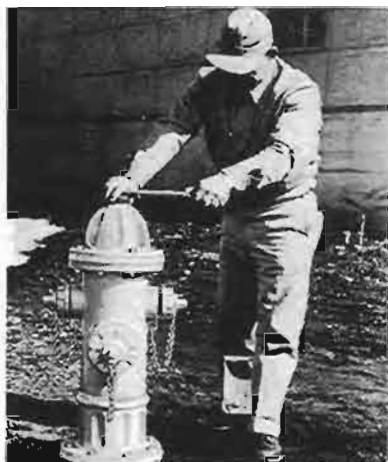
2a. Turn operating nut in opening direction until free of stem.
