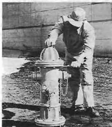
7. Replace bonnet. Turn operating nut in closing direction to engage stem. If bonnet has filler plug, make sure that the filler plug hole is aligned with the offset portion of the oil reservoir. Bolt in place.
