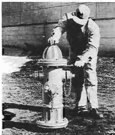
5a. Replace bonnet. Turn operating nut in closing direction to engage stem. Bolt in place.
