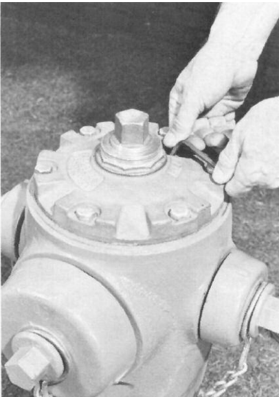
2. Remove the Oil Filler Plug and check the oil level. Oil should be level with the Oil Filler Plug hole.
