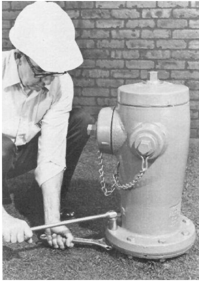
1. Loosen Nuts on Safety Flange Bolts.
