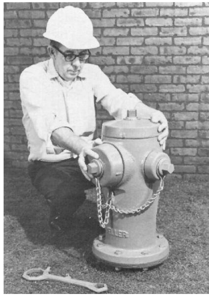
3. Rotate upper barrel section as desired.
