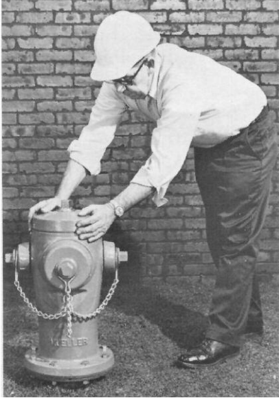
1. Remove the Weather Cap from the Hydrant.
