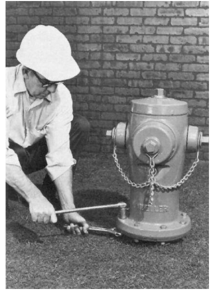
5. Tighten Safety Flange Bolts.
