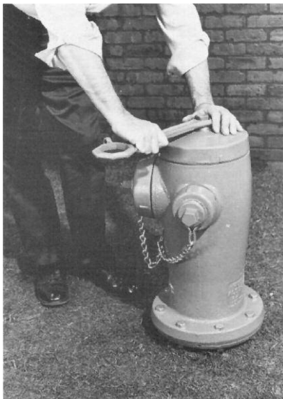
2. Turn Operating Nut slightly in the opening direction to relieve compression between barrel sections.
