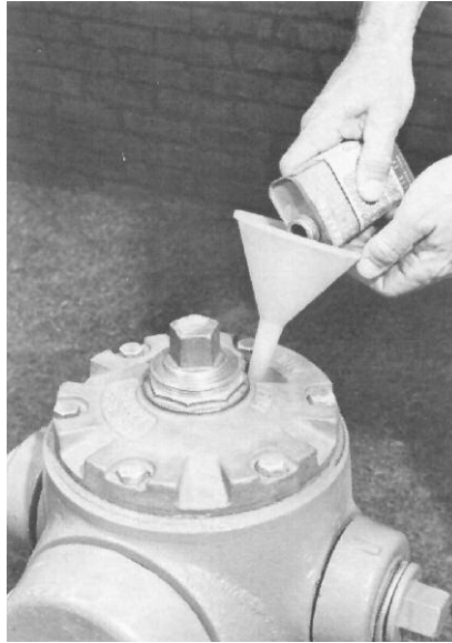
3. If oil is low, use a small funnel and add MUELLER Hydrant Lubricant.
