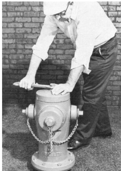
4. Tighten Operating Nut, turning in closing direction.
