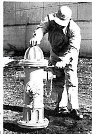
One man can put the hydrant back in service in a few minutes.
