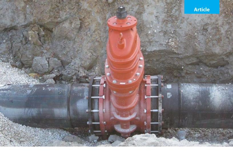
[stem] position is always preferred," advised Petito. "Provision for efficient and easy manual operation of the valves is also critical." [See #6].
