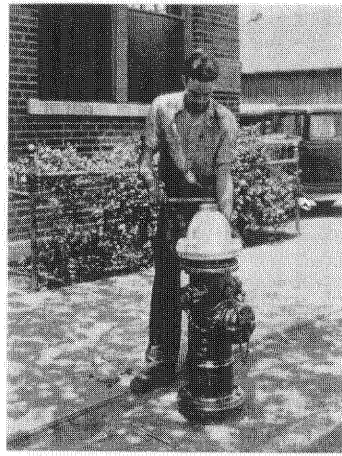
2. Turn Operating Nut in opening direction until free of Stem.
