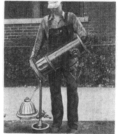
5. Holding gasket in position on flange, place upper barrel in position concentric with lower barrel.
