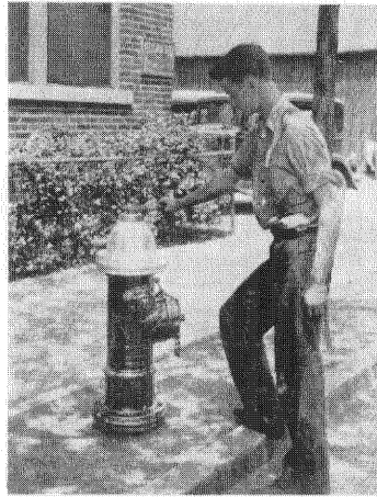
2. Turn Operating Nut slightly in opening direction to relieve friction between Barrel Sections.
