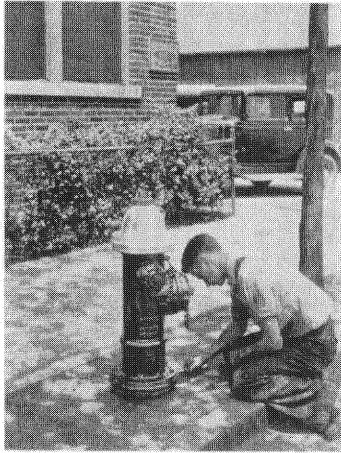
1. Loosen Nuts on Safety Flange Bolts.
