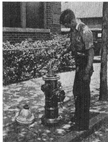
4. Replenish MUELLER-COLUMBIAN Hydrant Lubricant if necessary to within three-quarters of an inch from top of oil reservoir.
