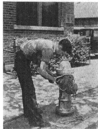
5. Replace Bonnet. Turn Operating nut to engage stem. Bolt in place.
