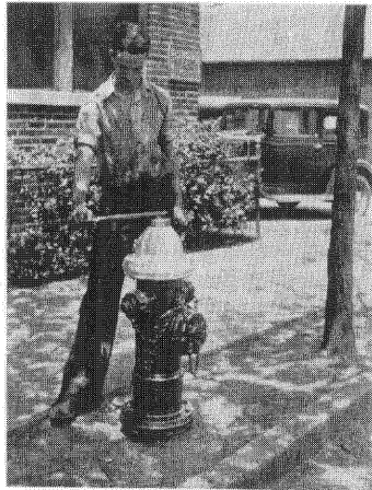
4. Tighten Operating Nut to closed position.
