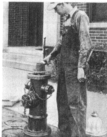
7. Bolt stuffing box assembly to upper barrel and tighten down stuffing box. Pour MUELLER-COLUMBIAN Hydrant Lubricant into oil reservoir until three-quarters of an inch from top.
