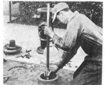
3. Screw new Safety Coupling down on to lower stem as far as threads permit. Screw upper stem into Safety Coupling until it contacts with lower stem.
