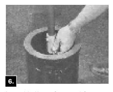
Assemble Upper Stem and Stem Coupling onto Extension Stem and retain it with Stainless Steel Clevis Pin and Reusable Clip.
