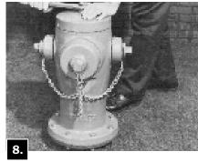
Remove the Oil Filler Plug in Housing. Pour Mueller Hydrant Lubricating Oil into oil reservoir until it is level with Oil Filler Plug hole. Replace Oil Filler Plug and Weather Cap. Open Hydrant fully. Tighten the Hose Nozzle Cap when water starts flowing and check all gaskets for leaks. Turn Operating Nut to fully closed position and remove Hose Nozzle Cap to allow Barrel to drain. Replace Hose Nozzle Cap.
