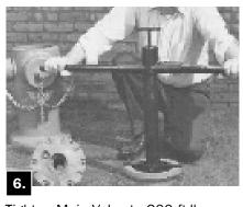
Tighten Main Valve to 200 ft-lbs. Turn on water at the Gate Valve and remove Wrench from Stem by removing Clevis Pin.
