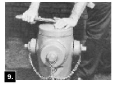
Unscrew one Hose Nozzle Cap slightly to bleed air. Open Hydrant fully. Tighten Hose Nozzle Cap when water starts flowing and check all gaskets for leaks. Turn Operating Nut to fully closed position and remove Hose Nozzle Cap to allow Barrel to drain. Replace Hose Nozzle Cap.
