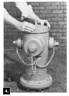
Replace the Oil Filler Plug and the Weather Cap.
