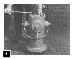
Remove Weather Cap, Hold Down Nut, Operating Nut and Anti-Friction Washer. Lubricate Brass Sleeve and slide over threaded stem end to prevent O-ring damage. Unbolt and remove Housing. Remove Brass Sleeve.
