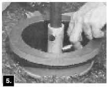
Assemble Upper Stem and new Stem Coupling onto Lower Stem and retain with new Stainless Steel Clevis Pin and new Reusable Clip furnished with Stem Coupling.
