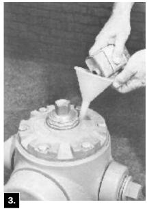
If oil is low, use a small funnel and add Mueller Hydrant Lubricant.
