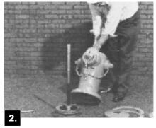
Remove Upper Barrel. Remove Upper Stem and Stem Coupling from Lower Stem. Slide slotted end of Wrench over Lower Stem. Align holes in Wrench and Stem and attach Wrench to Stem with a Clevis Pin. Lower Support Arm onto the flange of Lower Barrel and tighten Thumb Screw to hold Main Valve in the closed position. Shut off water at the Gate Valve.
