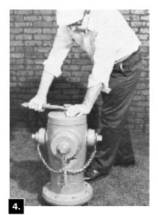
Tighten Operating Nut, turning in closing direction.
