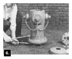
Place Flange Gasket on exposed Flange of Lower Barrel. Place Upper Barrel carefully in position on Lower Barrel. Be sure that it is concentric with Lower Barrel and that Gasket is centered. Bolt into place the two halves of Traffic Flange (with bevel on outer edge downward) and with Traffic Flange snugly fitting around Lower Barrel.
