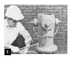
Attach Upper Barrel to Extension Barrel with Traffic Flange halves (with bevel on outer edge downward) and Bolts, being sure Traffic Flange Gasket is in place.
