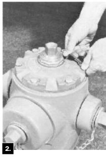
Remove the Oil Filler Plug and check the oil level. Oil should be level with the Oil Filler Plug hole.
