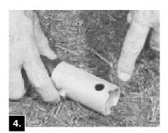
Place Extension Stem and Extension Coupling on Lower Stem and retain it with Stainless Steel Clevis Pin and Reusable Clip.
