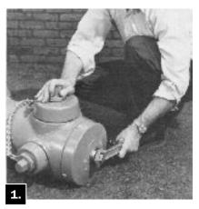
Tighten Operating Nut to be sure Main Valve is in the fully CLOSED position.
