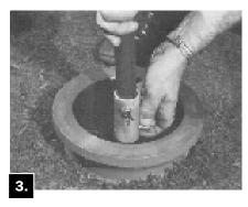
Remove the Upper Barrel and remove Stem and Stem Coupling by removing the lower Stainless Steel Reusable Clip and Clevis Pin.
