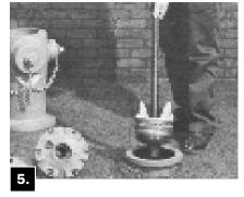
Lower Main Valve assembly and carefully thread Seat Ring into the base of the Hydrant hand tight. Raise the Main Valve leaving about 1/2" of play between the Main Valve and Seat. Lower Support Arm onto flange of Lower Barrel and tighten Thumb Screw.
