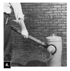
Lubricate O-ring on new Nozzle. Screw new Nozzle in place hand tight and place Nozzle Wrench behind threaded section of Nozzle so that Wrench gaps engage Nozzle drive lugs. Screw on Nozzle Cap to hold the Wrench in place. Attach a length of pipe to handle of Nozzle Wrench and tighten.
