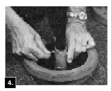
Place Extension Stem and Extension Coupling on Lower Stem and retain it with Stainless Steel Clevis Pin and Reusable Clip.
