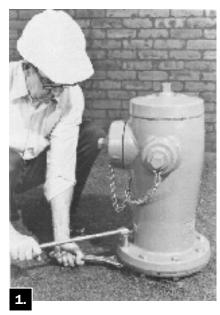
Loosen Nuts on Traffic Flange Bolts.
