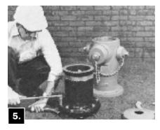
Attach Extension Barrel to Lower Barrel with solid Flange halves (without groove) and Bolts, being sure Flange Gasket is in place.
