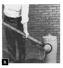
Attach a length of pipe over handle end of Wrench and unscrew the Nozzle.
