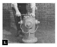
Remove the Weather Cap, Hold Down Nut, Anti-Friction Washer and Operating Nut from the Hydrant. Lubricate outside of Brass Sleeve and slide over threaded stem to prevent O-ring damage. Unbolt and remove the Housing. Remove Brass Sleeve.
