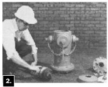
Slide slotted end of Wrench over top of Stem and engage the slot with Pin welded to Upper Stem. Tighten "T" handle of Wrench firmly. Lower support arm onto top of Upper Barrel and tighten Thumb Screw to hold the Main Valve in the closed position. Shut off water at the Gate Valve. Remove Main Valve assembly by turning Seat Wrench counter-clockwise.
