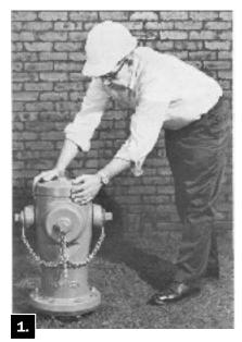
Remove the Weather Cap from the Hydrant.
