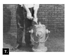
Attach the Brass Sleeve to Upper Stem and lubricate outside to protect O-rings from thread damage. Place Housing onto Upper Barrel and tighten Bolts. Remove Brass Sleeve, reassemble Operating Nut, Anti-Friction Washer and Hold Down Nut.\* Be sure O-ring Seals are in good condition at thread shoulder on outside of Hold Down Nut and on inside where contact is made with Operating Nut.
