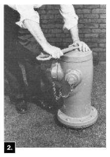
Turn Operating Nut slightly in the opening direction to relieve compression between barrel sections.
