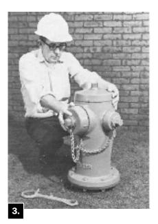
Rotate upper barrel section as desired.
