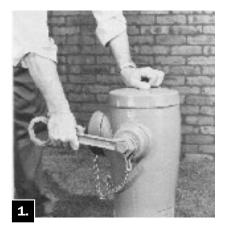
Unscrew and remove the Nozzle Cap. Using a pointed tool or awl, remove the Nozzle Lock. If Nozzle is retained with retaining screw, use screwdriver to remove screw.
