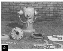
Remove Stainless Steel Reusable Clip from Stainless Steel Clevis Pin. Remove the Clevis Pin and damaged Stem Coupling from Upper Stem. Unbolt and remove broken Traffic Flange from Upper Barrel. Remove Weather Cap, Hold Down Nut, Anti-Friction Washer and Operating Nut from Upper Barrel. Lubricate Brass Sleeve and slide over threaded Stem end to prevent O-ring damage. Unbolt and remove Housing. Remove Upper Stem from Housing.
