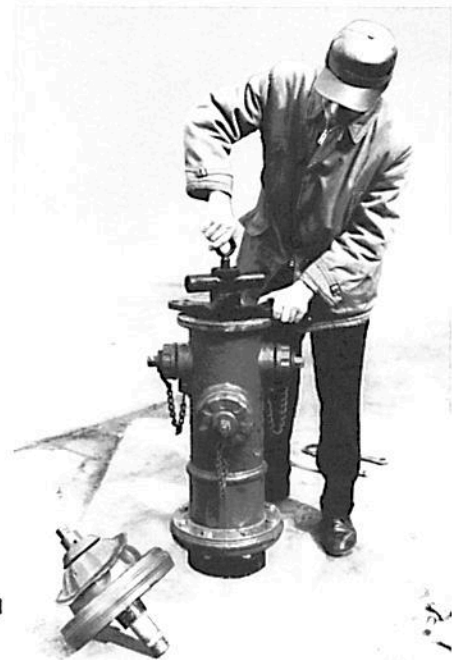
3 Next, attach the Seat Removal Wrench
