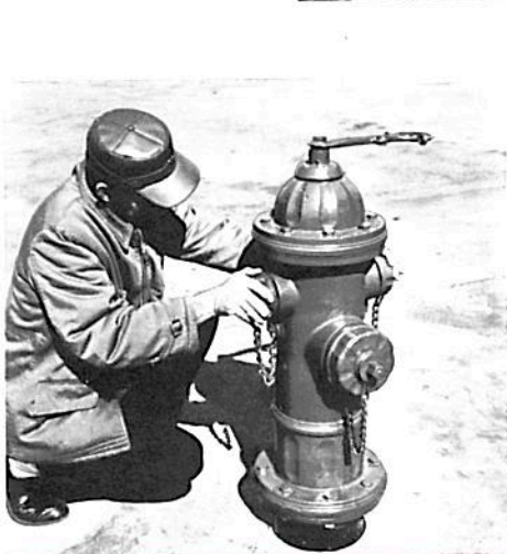
The upper barrel can be rotated to permit nozzles to be faced in any desired direction. (Not in a specific number of positions such as 4, 6, or 8).
