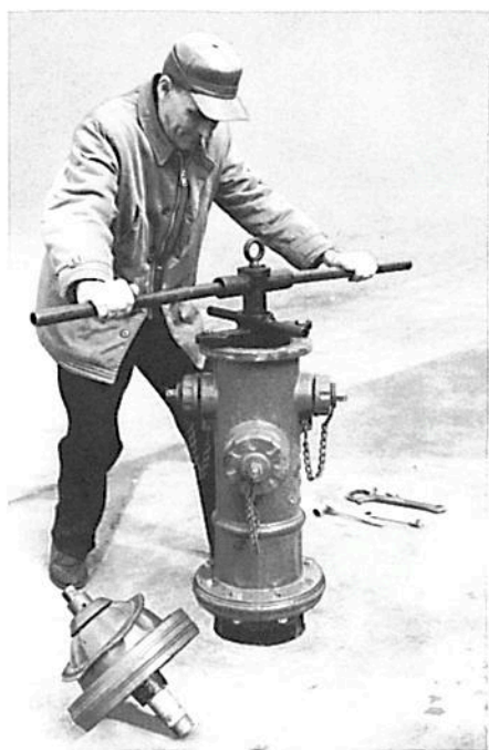
4 Remove main valve and seat ring
