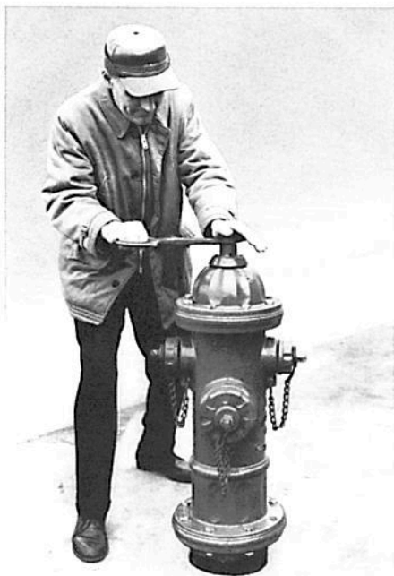
1 First Isolate the hydrant
