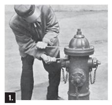
Remove Bonnet Bolts and Nuts. Rotate Operating Nut in opening direction to fully opened position. This lifts Bonnet off the Upper Barrel. Rotate bonnet assembly counter-clockwise to detach Bonnet from Upper Stem threads. Lift off Bonnet, remove Bonnet Gasket.
