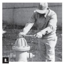
Replace Hold Down Nut\* being sure O-ring seals are in good condition at thread shoulder on outside of Hold Down Nut and on inside where contact is made with Operating Nut. Replace Weather Cap. Tighten Bonnet Bolts. Check gasket tightness by opening one hose cap slightly before opening Hydrant to bleed air. Open Hydrant until barrel fills with water, tighten Hose Cap, open Hydrant fully. Check gaskets, and then turn Operating Nut to fully closed position.
