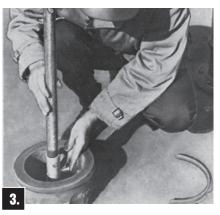
Place Extension Stem and Extension Coupling on Lower Stem and retain it with stainless steel Clevis Pin and stainless steel Cotter Pin.
