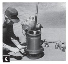
Attach Extension Barrel to Lower Barrel with solid flange halves and bolts, being sure Flange Gasket is in place (tighten bolts to 1,000 in-lbs).
