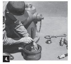
Place Extension Stem and Extension Coupling on Lower Stem and retain it with stainless steel Clevis Pin and stainless steel Cotter Pin.
