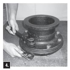
Attach Extension Barrel to Lower Barrel with solid Flange halves (without groove) and Bolts, being sure O-ring is in place.
