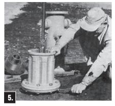
Attach Extension Barrel to Lower Barrel with solid Flange Halves (without groove) and bolts, being sure Flange Gasket is in place.
