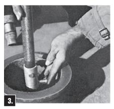
Place Extension Stem and Extension Coupling on lower stem and retain it with stainless steel Clevis Pin and stainless steel Cotter Pin.
