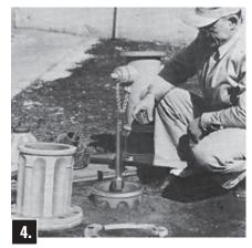
Screw Extension Stem into Extension Coupling until it contacts Lower Stem. Align tongue and groove of stems with hole in Extension Stem Coupling. Screw Extension Stem Coupling upward until tongue and groove of stems firmly lock together. Tighten with wrench, then, screw in Set Screw in Extension Stem Coupling.
