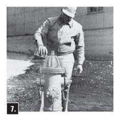
Check Bonnet Gasket. Attach the A-366 Brass Sleeve, if it had been removed, to Upper Stem and lubricate outside to protect O-ring seals from thread damage. Place Bonnet onto Upper Barrel and assemble Bonnet Bolts only hand tight. Remove Brass Sleeve. Reassemble Operating Nut and remove Oil Plug in side of Bonnet. Pour Mueller Hydrant Lubricant into Oil Reservoir until it is filled to the level of the Oil Plug. Replace Oil Plug.
