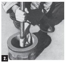
Unbolt Traffic Flange and remove Upper Barrel. Remove Upper Stem and Stem Coupling by removing the lower stainless steel Cotter Pin and stainless steel Clevis Pin.
