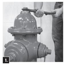
Remove Hold-Down Nut, Anti-Friction Washer and Operating Nut from Bonnet. Lubricate outside of Brass Sleeve and slide over threaded stem end to prevent O-ring damage. Unbolt Bonnet from Upper Barrel and remove. Remove Brass Sleeve.
