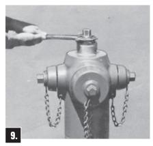
Tighten Hold Down Nut to 100 ft-lbs and bend Lock Washer Ears over Hold Down Nut flats in two places and over Operating Housing in two places.
