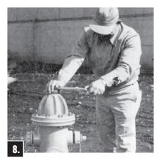
Replace Hold Down Nut\* being sure O-ring seals are in good condition at thread shoulder on outside of Hold Down Nut and on inside where contact is made with Operating Nut. Replace Weather Cap. Tighten Bonnet Bolts. Check gasket tightness by opening one hose cap slightly before opening Hydrant to bleed air. Open Hydrant until barrel fills with water, tighten Hose Cap, open Hydrant fully. Check gaskets, and then turn Operating Nut to full closed position.
