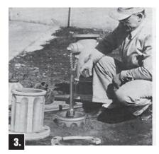
Screw Extension Stem into Extension Coupling until it contacts Lower Stem. Align tongue and groove of stems with hole in Extension Stem Coupling. Screw Extension Stem Coupling upward until tongue and groove of stems firmly lock together. Tighten with wrench, then screw in set screw in Extension Stem Coupling.
