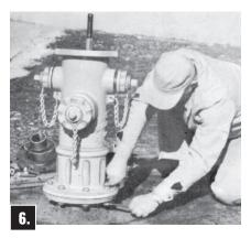
Attach Upper Barrel to Extension Barrel with Traffic Flange Halves (with groove) and bolts, being sure Flange Gasket is in place.
