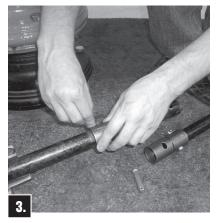
Place Extension Stem and Extension Coupling on Lower Stem and retain it with stainless steel Clevis Pin and stainless steel Cotter Pin.
