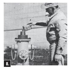
Check Stuffing Box Gasket. Lubricate A-366 Brass Sleeve. Slide Sleeve over threaded area of stem to protect O-rings from damage by threads. Place Stuffing Box in position and bolt to barrel. Remove Brass Sleeve. Pour Mueller Hydrant Lubricant into Oil Reservoir until <sup>3</sup>/<sub>4</sub>" from top.
