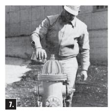
Check Bonnet Gasket. Attach the A-24099 Brass Sleeve, if it had been removed, to Upper Stem and lubricate outside to protect O-ring seals from thread damage. Place Bonnet onto Upper Barrel and assemble Bonnet Bolts only hand tight. Remove Brass Sleeve. Reassemble Operating Nut and remove Oil Plug in side of Bonnet. Pour Mueller Hydrant Lubricant into Oil Reservoir until it is filled to the level of the Oil Plug. Replace Oil Plug.
