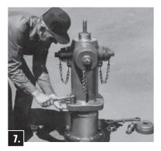
With lubricated Brass Sleeve on threads of Upper Stem and Upper Barrel Seal in position, lift Upper Barrel over Upper Stem and onto extension section Attach Traffic Flange Clips and Traffic Flange Clip Bolts loosely, face nozzles in desired position and tighten Traffic Flange Clip Bolts uniformly to 1,000 in-lbs.
