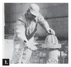
Remove Weather Cap, Hold Down Nut and Operating Nut from Bonnet. Lubricate A-366 Brass Sleeve and slide over threaded stem end to prevent O-ring damage. Unbolt Bonnet from Upper Barrel and remove. Remove Brass Sleeve.
