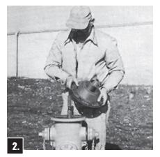
Remove four bolts in stuffing box. Lubricate A-366 Brass Sleeve. Slide Sleeve over threaded area of stem to protect O-rings from damage by threads. Lift stuffing box off carefully. Remove Brass Sleeve.
