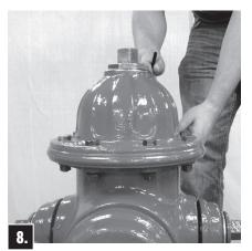
Remove Oil Filler Plug in side of Bonnet. Pour MUELLER Hydrant Lubricant into Oil Reservoir until it is level with Oil Filler Plug Hole. Replace Oil Filler Plug (see Lubrication section on page 8).
