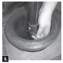
Assemble Upper Stem and Stem Coupling onto Extension Stem and retain it with stainless steel Clevis Pin and stainless steel Cotter Pin.
