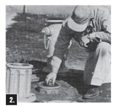
Unbolt Traffic Flange and remove Upper Barrel. Unscrew set screw in Sleeve.
