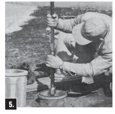
Place new Stem Coupling Sleeve part onto Upper Stem. Screw new Stem Coupling part onto Lower Stem as far as threads permit.
