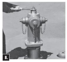
With extension section and Hydrant securely bolted in place, remove Brass Sleeve, replace Operating Nut, Lock Washer, and Hold Down Nut.
