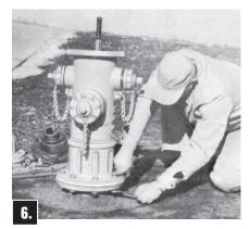
Attach Upper Barrel to Extension Barrel with Traffic Flange Halves (with groove) and bolts, being sure Flange Gasket is in place.
