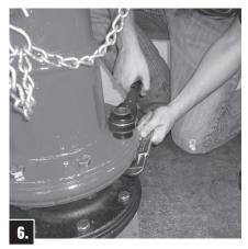
Attach Upper Barrel with Traffic Flange Halves (with bevel on outer edge downward) and Bolts; being sure Traffic Flange O-ring\* is in groove in Upper Barrel. Tighten Bolts to 60 ft-lbs.
