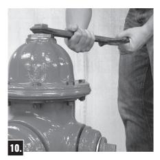
Turn Operating Nut in closing direction to make sure Main Valve is closed tightly, then turn in opening direction approximately 1/4 turn to relieve tension on operating mechanism.
