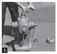
Remove Weather Cap, Hold Down Nut, Lock Washer and Operating Nut. Put on Brass Sleeve and lubricate to protect O-rings in operating housing.
