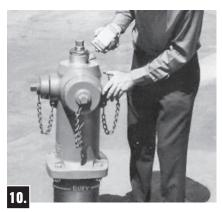
Remove Oil Filler Plug and add Mueller<sup>®</sup> Hydrant Lubricant until level with Filler Plug hole. Replace Oil Filler Plug and replace Weather Cap.
