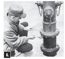
Attach Upper Barrel to Extension Barrel with Traffic Flange halves (with groove) and bolts, being sure Traffic Flange Gasket is in place.
