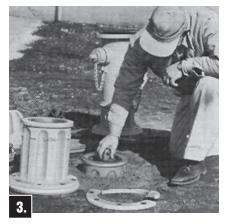
Unbolt Traffic Flange and remove Upper Barrel.
