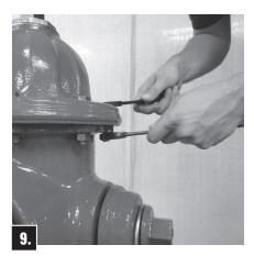
Torque Bonnet Bolts to 40-80 ft-lbs. Torque Hold-Down Nut to 200-300 ft-lbs. after Bonnet Bolts are tight. Open Gate Valve. Unscrew one Hose Nozzle Cap slightly to bleed air. Open Hydrant fully. Tighten Hose Nozzle Cap when water starts flowing and check all flange connections for leaks. Turn Operating Nut to fully closed position and remove Hose Nozzle Cap to allow Barrel to drain. Replace Hose Nozzle Cap.
