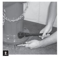
Unbolt Traffic Flange. Remove Upper Barrel. Remove Upper Stem and Stem Coupling by removing the lower stainless steel Cotter Pin and stainless steel Clevis Pin.
