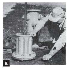
Attach Extension Barrel to Lower Barrel with solid Flange Halves (without groove) and bolts, being sure Flange Gasket is in place.
