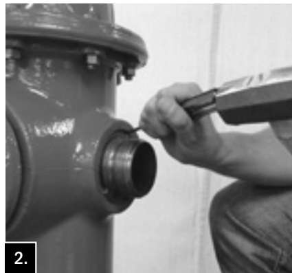
Remove stainless steel Nozzle Lock by driving it out with a pointed tool and hammer.
