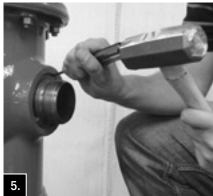
Remove Nozzle Cap and Nozzle Wrench. Place the Nozzle Lock (Part 143137), lengthwise in the slot formed by the Nozzle Drive Lugs and the Barrel Bore. Drive the A-316 Nozzle Lock in place by striking the Nozzle Lock Installation Tool several times with a heavy brass hammer.
