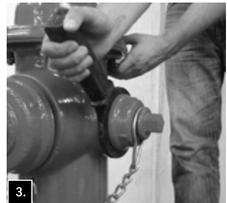
Place A-316 Nozzle Wrench on Nozzle with Wrench Forks facing toward Hydrant Barrel and locked onto Nozzle Drive Lugs. Replace Nozzle Cap and tighten until Cap rests loosely against backside of Wrench. Remove Nozzle (nozzle threads out in a clockwise rotation). Additional leverage may be obtained by placing a length of 2" schedule 40 steel pipe over the handle of the Nozzle Wrench.
