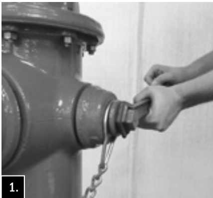
Remove Nozzle Cap.
