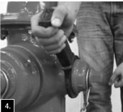
Install Nozzle O-ring on the inlet side of the Nozzle. Thread new Nozzle into Upper Barrel, attach Nozzle Wrench as described in Step 3, and tighten Nozzle (nozzle threads in a clockwise rotation) to approximately 600 ft-lbs torque (100 lbs pull on a 6' lever).
