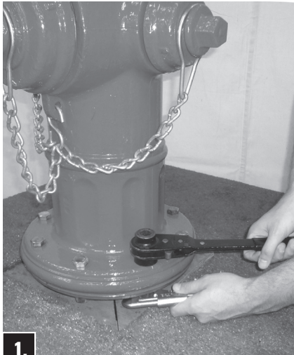
1. Loosen Nuts on Traffic Flange Bolts.
