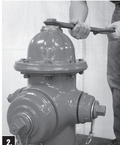
2. Turn Operating Nut slightly in the opening direction to relieve compression between Barrel sections.
