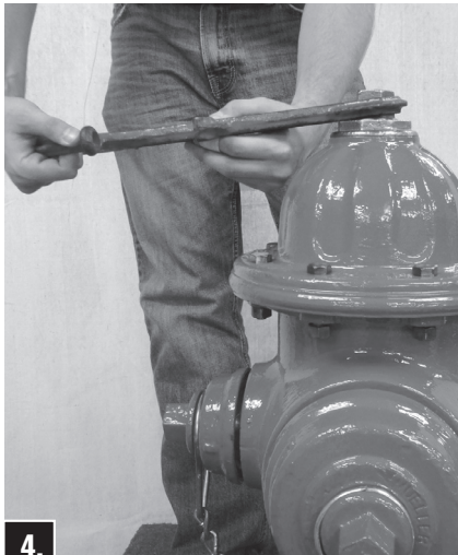
4. Tighten Operating Nut, turning in closing direction.
