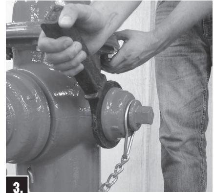
3. Place A-316 Nozzle Wrench on Nozzle with Wrench Forks facing toward Hydrant Barrel and locked onto Nozzle Drive Lugs. Replace Nozzle Cap and tighten until Cap rests loosely against backside of Wrench. Remove Nozzle (nozzle threads out in a clockwise rotation). Additional leverage may be obtained by placing a length of 2" schedule 40 steel pipe over the handle of the Nozzle Wrench.
