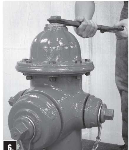
6. Turn Operating Nut in closing direction to make sure Main Valve is closed tightly, then turn in opening direction approximately 1/4 turn to relieve tension on operating mechanism.
