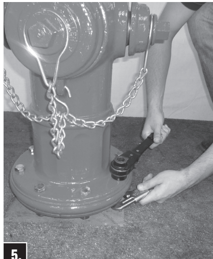
5. Tighten Traffic Flange Bolts to 60 ft-lbs.
