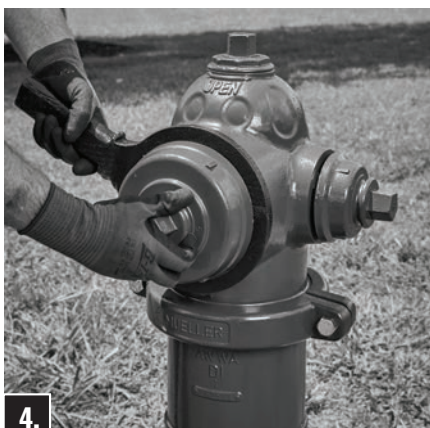
4. Replace Nozzle Cap and tighten until Cap rests loosely against backside of Wrench. Remove Nozzle (nozzle threads out in a clockwise rotation). Additional leverage may be obtained by placing a length of 2" schedule 40 steel pipe over the handle of the Nozzle Wrench. Install Nozzle O-ring on the inlet side of the Nozzle. Thread new Nozzle into Upper Barrel, attach A-316 Nozzle Wrench as described in Step 3, and tighten Nozzle (nozzle threads in a clockwise rotation) to approximately 600 ft-lbs torque (100 lbs. pull on a 6' lever).
