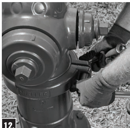
12. Tighten Nozzle Section Clamp Bolts (2) to 70-130 ft-lbs.
