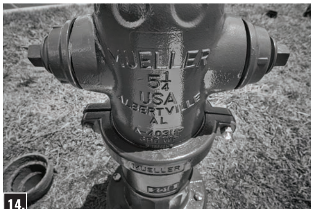
14. Loosen one Hose Nozzle Cap and turn Operating Nut in the open direction until water can be seen. Tighten hose cap and check Nozzle Section Clamp for leaks.
