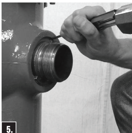
5. Remove Nozzle Cap and A-316 Nozzle Wrench. Place the Nozzle Lock (Part 143137), lengthwise in the slot formed by the Nozzle Drive Lugs and the Nozzle Section Bore. Drive the Nozzle Lock in place by striking the Nozzle Lock Installation Tool (Part 143132) several times with a heavy brass hammer.
