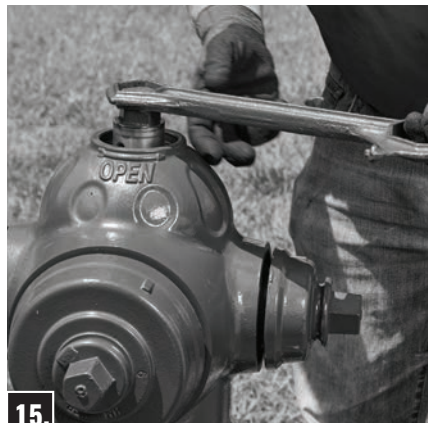
15. Turn Operating Nut in closing direction to make sure Main Valve is closed tightly, then turn in opening direction approximately 1/4 turn to relieve tension on operating mechanism.
