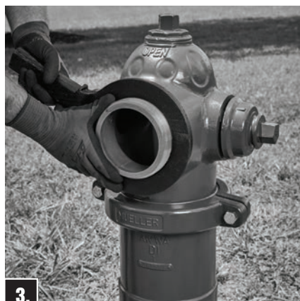
3. Place Nozzle Wrench, A-316, on Nozzle with Wrench Forks facing toward Hydrant Barrel and locked onto Nozzle Drive Lugs.
