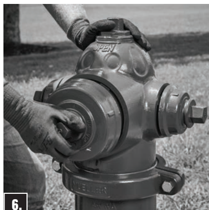
6. Replace and tighten Nozzle Cap.
