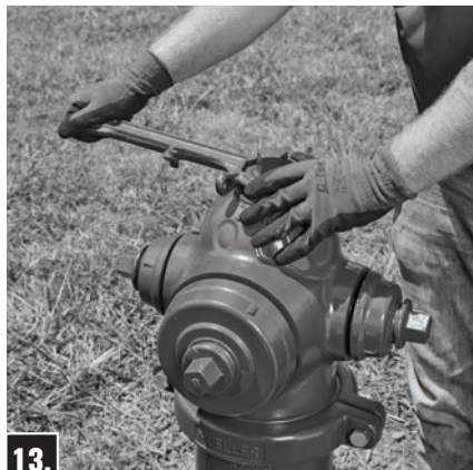
13. Torque Hold-Down Nut to 200-300 ft-lbs after Nozzle Section Clamp Bolts (2) are tight.
