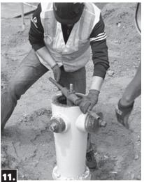
11. Before lowering completed rod assembly into hydrant, check seat gasket and lubricate with manufacturer approved NSF food-grade grease. Using seat wrench, turn clockwise to seat lower rod.
