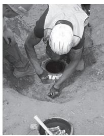
**4.** Undo bolts and nuts and remove upper barrel, traffic flange and barrel gasket. (Do not discard nuts and bolts; they are needed for Step 8).
