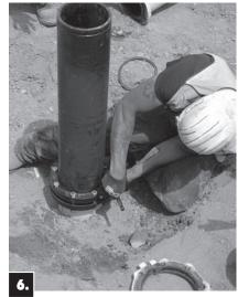
**6.** Install extension to lower barrel using barrel bolts and ground flange nuts (ID-11 and ID-9). See torque specification values on page 6.
