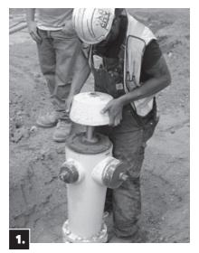
1. To remove bonnet, locate the bonnet pins that are directly above the hose caps. Using hammer and punch, drive the pins into the housing. (Do not discard bonnet pins; they are needed for final bonnet assembly in Step 13).
