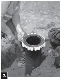
**7.** Reinstall the traffic flange using side bolts and nuts (ID-6 and ID-7) as well as barrel gasket (ID-10).
