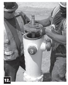
**12.** Install new housing gasket (ID-12) to the housing assembly and carefully reinstall housing over the top rod (turn in opposite direction of Step 2). Replace bolts in bearing housing by installing the longer bolts first, then the 2 short bolts in the recessed pockets (reverse of Step 2).
