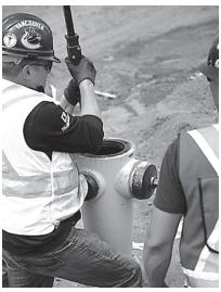
**3.** Using the seat removal wrench, turn counter-clockwise to remove the lower rod and seat assembly.
