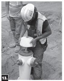
**13.** Reinstall bonnet using bonnet pins previously removed in Step 1.
