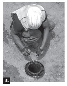
**5.** Install the D.I. flange (ID-5) flat side down, using side bolts and nuts (ID-6 and ID-7) to lower barrel. Then, place the new barrel gasket (ID-10) on the lower barrel.
