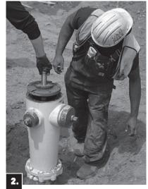
2. Starting with the 2 short bolts in the recessed pockets, remove all 6 housing bolts and turn the operating nut counterclockwise for Open Left Hydrants or clockwise for Open Right Hydrants. After operating nut has been disengaged from the top rod, lift housing carefully to remove from the hydrant. (Do not discard bolts; they are needed for Step 12).
