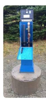
Water Authority, sampling was previously done inside of homes, businesses, and on hydrants. Portugal Cove-St. Philip's recently installed this Hydro-Guard blow-off sampling station (B.O.S.S.) to make water sampling easier, more consistent, and produce more reliable data.
