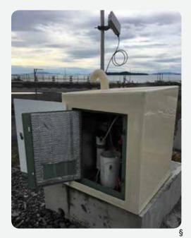
Located in Prince Rupert, British Columbia, Ridley Terminal serves as a shipping port for grain, coal and lumber to the U.S. and China. While there are several buildings on the property, the port has large water distribution lines with little demand which resulted in chlorine residuals of 0.5 ppm and less. After installing Hydro-Guard S.M.A.R.T. automatic flushing units, Ridley Terminal was able to resolve their low chlorine residual issue.
