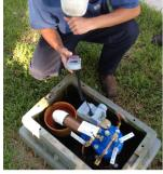
water sampling protocol, Groby assisted in designing and implementing a flush cycle that force-flushes 27 miles of the water distribution system.
