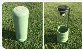
The City of Durham (North Carolina) is now using a pedestal enclosure mounting kit from Mueller Co. for Hydro-Guard remote pressure monitoring system installations in areas where groundwater levels are frequently near the top of a valve box. This approach elevates the remote telemetry unit above ground and out of standing water.
