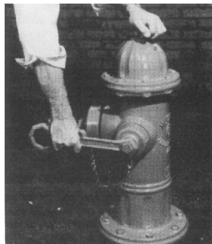
7. Replace and tighten Nozzle Cap.
