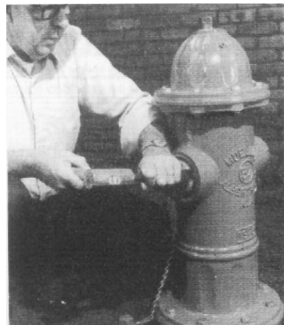
6. Remove Nozzle Cap and A-316 Nozzle Wrench. Place the Nozzle Lock (Part 143137), lengthwise in the slot formed by either of the Nozzle Drive Lugs and the Barrel Bore. Drive the Nozzle Lock in place by striking the Nozzle Lock Installation Tool (Part 143132) several times with a heavy brass hammer.
